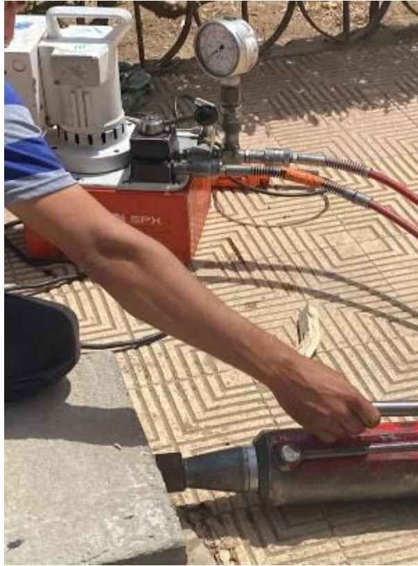
Fig. 3: Applying the post-tensioning force using a hydraulic jack
