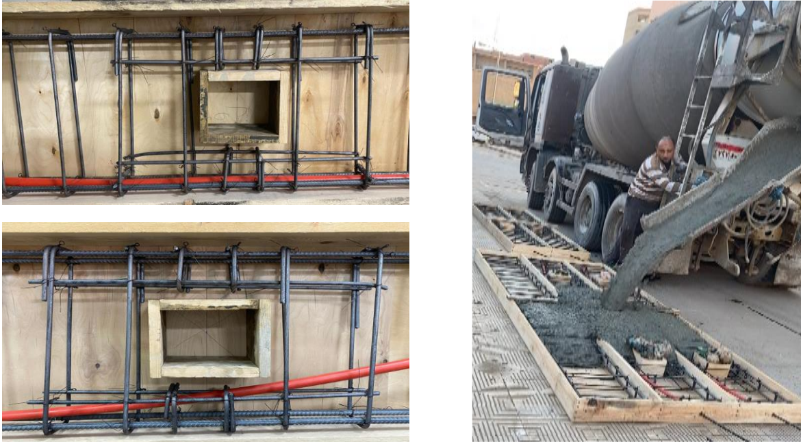
Fig. 2: Reinforcement details and casting of test beams using ready-mix concrete
