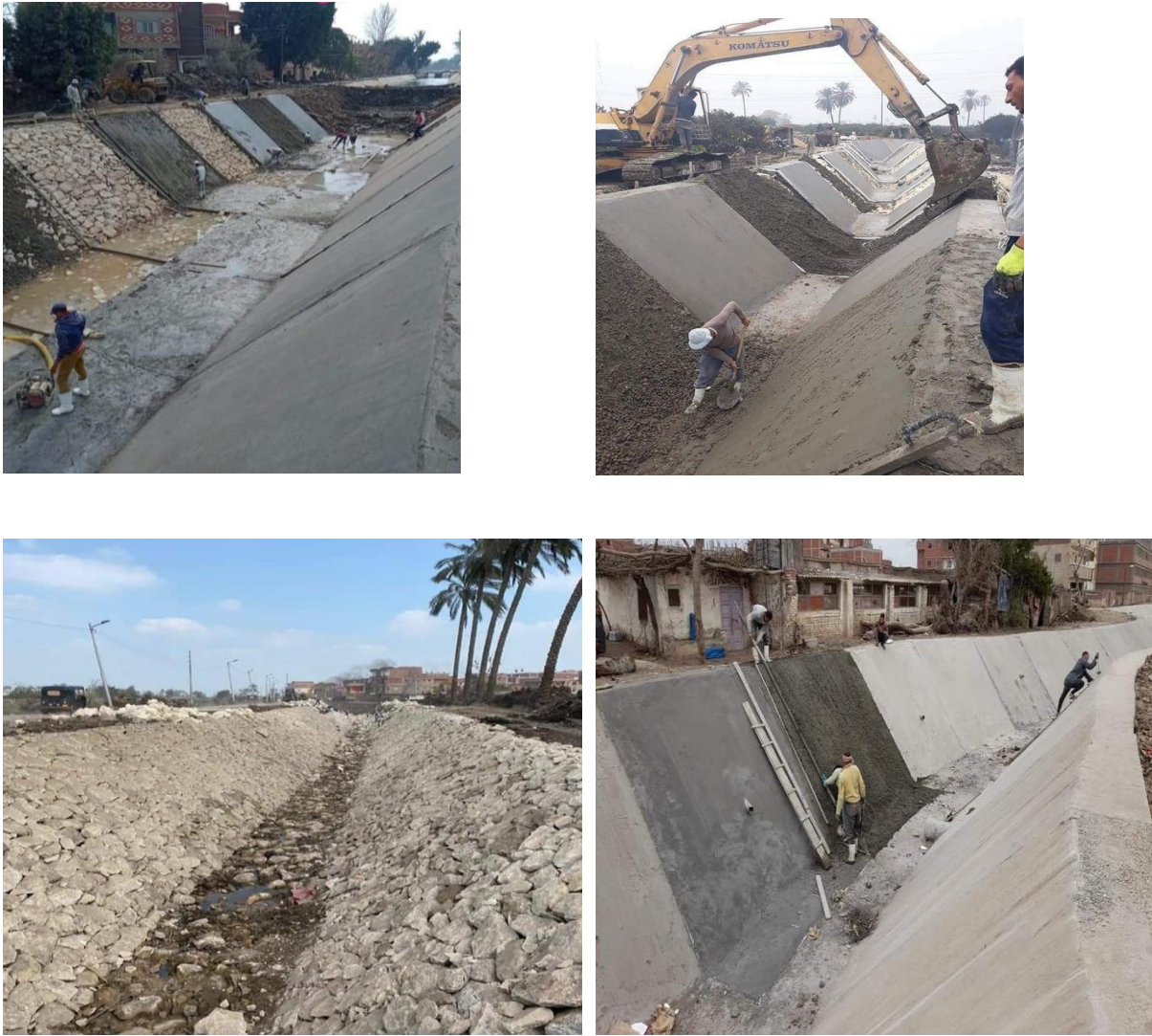
Fig. 5: Concrete lining for branch and distribution canals
