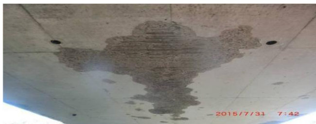
Fig. 7. Fire-damaged span 2.
