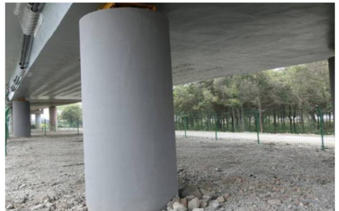
Fig. 27. Steel plate strengthening at the soffit.
