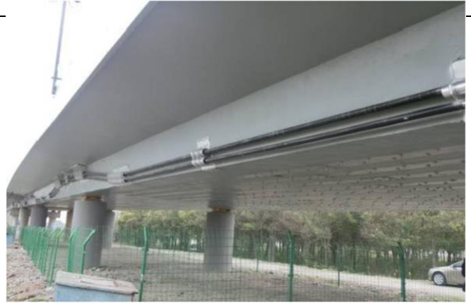
Fig. 26. External prestressing strengthening at webs.
