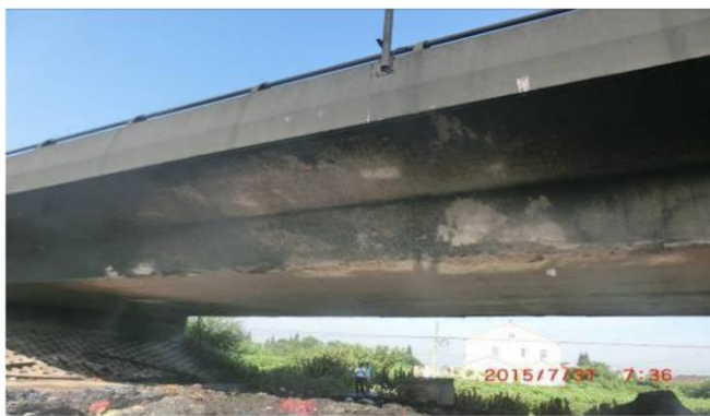
Fig. 6. Fire-damaged span 1.
