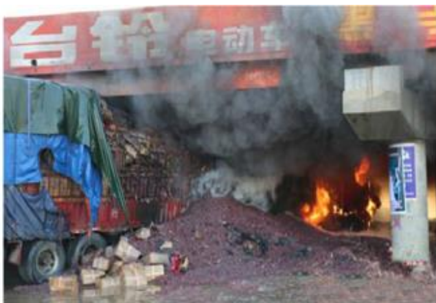
Fig. 2. Fire below the bridge span.
