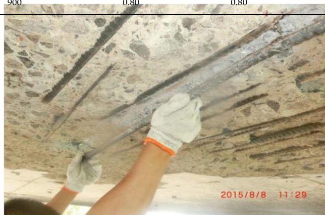
Fig. 11. Bar sample from the soffit.
