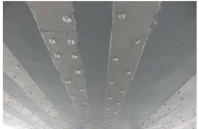
Fig. 27. Steel plate strengthening at the soffit.
